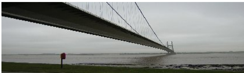
The Humber Bridge
